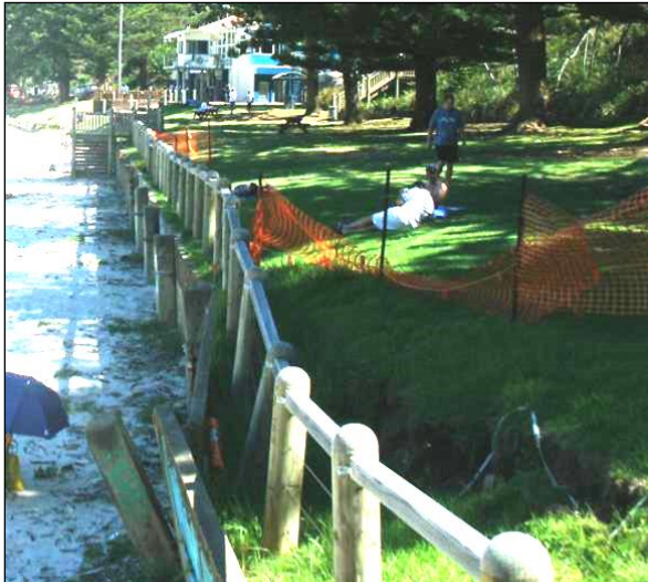
Figure 3-6 Movement of the precast panels and erosion behind the retaining wall at the northern end and Rocks placed along the southern end of the existing retaining wall
