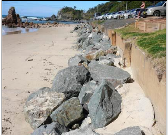
Figure 3-6 Movement of the precast panels and erosion behind the retaining wall at the northern end and Rocks placed along the southern end of the existing retaining wall
