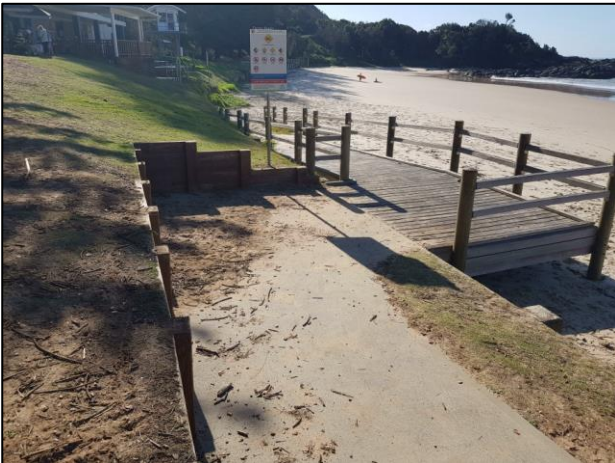
Figure 3-6 Movement of the precast panels and erosion behind the retaining wall at the northern end and Rocks placed along the southern end of the existing retaining wall
